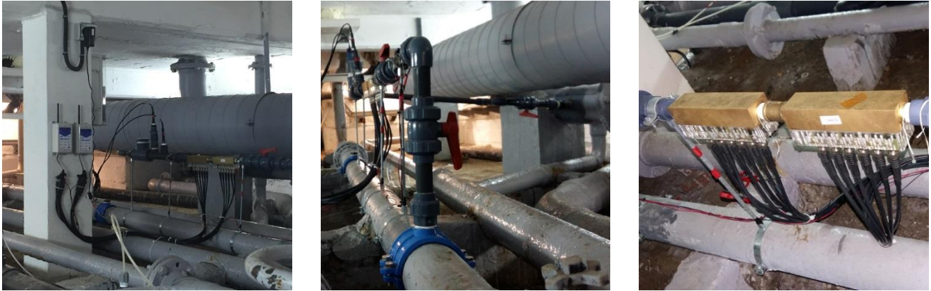
Figure 4. Two smart sensors from the wireless monitoring infrastructure
